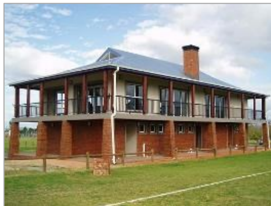
Montana High School Library in Worcester makes superb use of the natural insulating properties of clay brick. Photograph courtesy of Worcester Brick.
